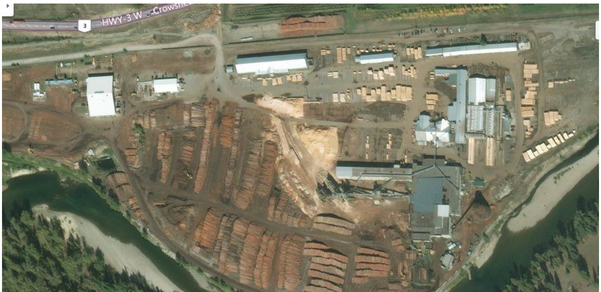
Figure 3 Vaagen Fiber Canada mill
