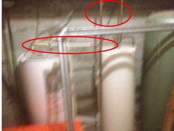
**Figure 2: Un-insulated piping**
