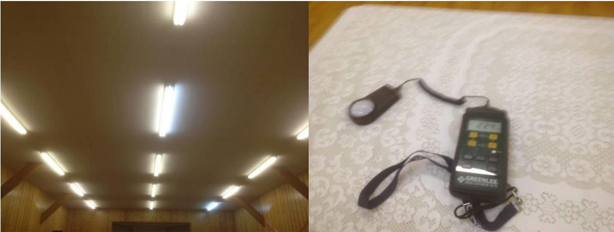
**Figure 4: T12 Lamps Requiring Replacement**
